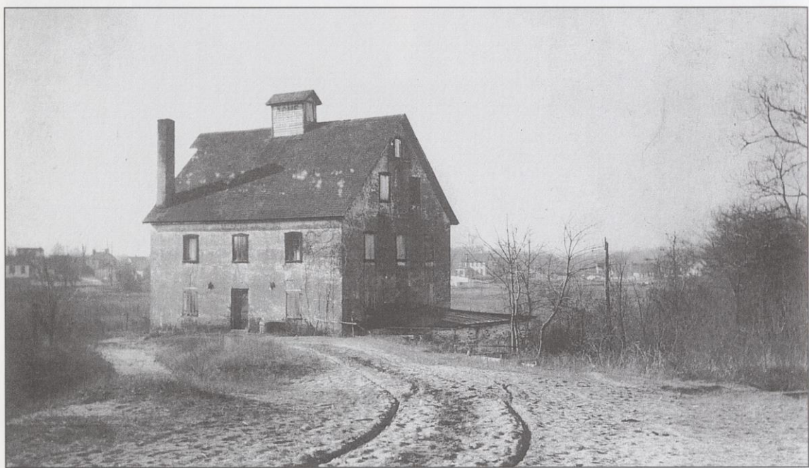
Avalon Mill was built by the Calvert family and was located in Bladensburg off Edmonston Road. It was torn down in 1929. (Submitted by Susan Reidy, historian for the Natural and Historical Resources Division of Maryland-National Capital Park & Planning Commission; courtesy of S.K. Cristofane.)
